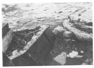
April 21, 1948, this wooden pier of the third span of the East Coulee C.P.R. bridge is starting to lose its metal plate protection from the damaging effects of the ice floes. The side metal plate is already gone, only the "V" shaped point is left remaining. Note: The piers were originally constructed of wooden pilings with a wooden framework around them. The centre area was filled with rocks as can be seen.
