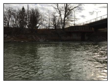
Photograph 9 Riprap armouring surrounding the abutments of the Highway 56 bridge, looking at the right (south) bank.
